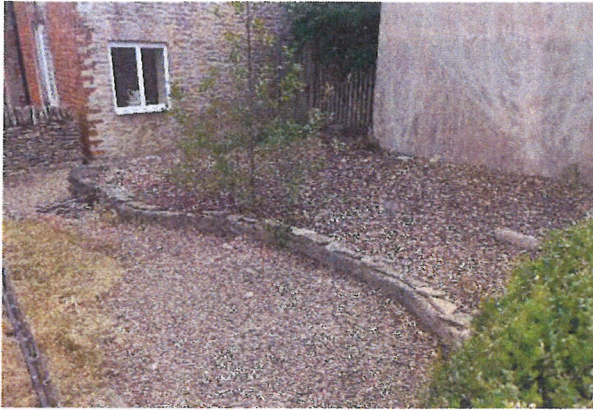
D-17 Dynevor Place: well on raised part of side-garden
