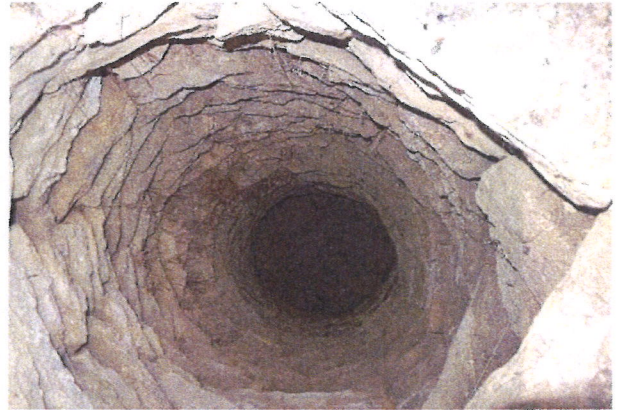
D-18 Dug-well interior at 2 Dynevor Place
