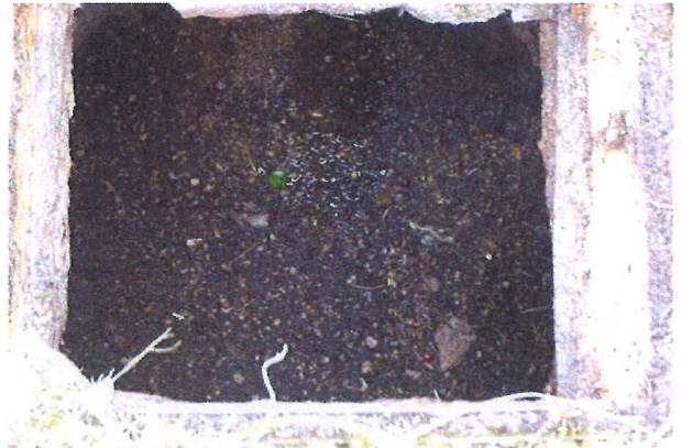
D-20 Dug-well at Manor Farm: interior backfilled
